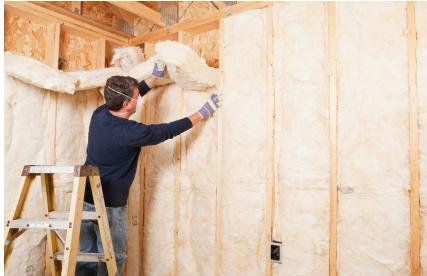
Insulation is material used in buildings to help to keep the heat inside to make them warmer.
